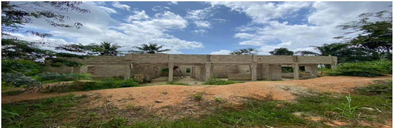
Figure 5: Completion of 1No CHPS Compound at Saman Abotar Park (On-going)
