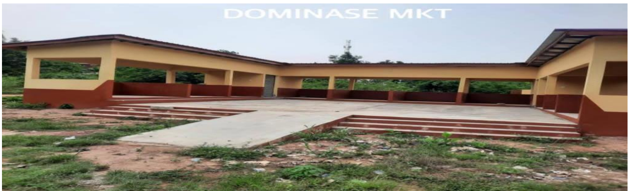
Figure 6: Completion of 1No. 12Unit Market sheds, 2No. Stores and Toilet Facility at Dominase
