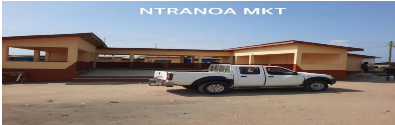
Figure 7: Completion of 1No. 12Unit Market sheds, 2No. Stores and Toilet Facility at Ntranoa
