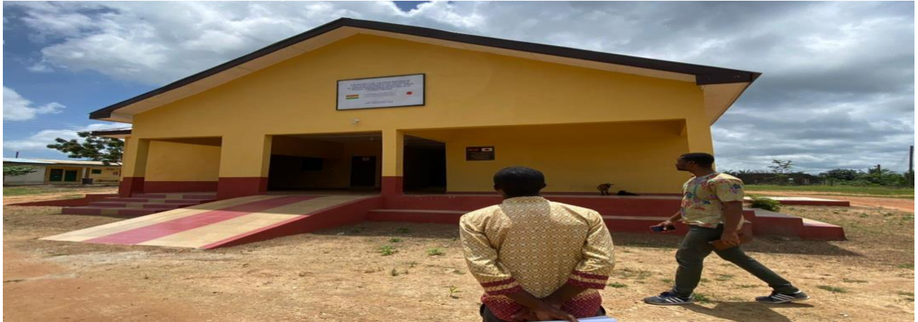
Figure 1: Fully Furnished CHPS Compound with Mechanized Borehole at Berase
