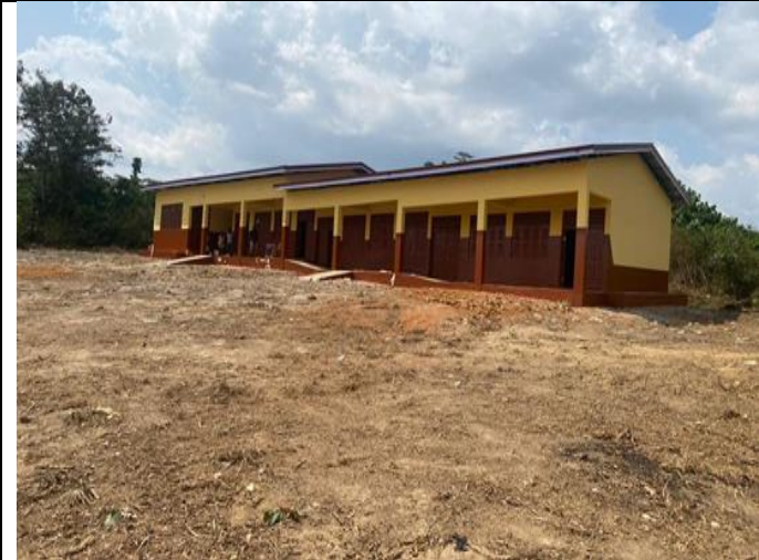
1. NO 3-UNIT CLASSROOM BLOCK WITH OFFICE & STORE WITH 150.NO MONO DESK, 4. NO OFFICE TABLES & CHAIR AT ESSIAM
