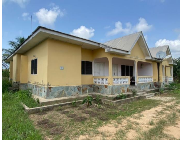
Renovation of Planning & Budget Flat
