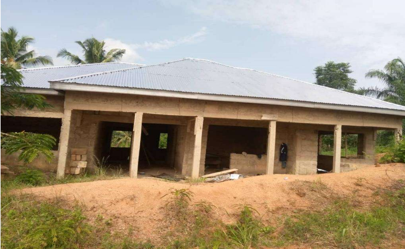
Figure 4: 1 No. CHPS Compound with Ancillary facilities at Saman, Abotar, Park (On-going)
