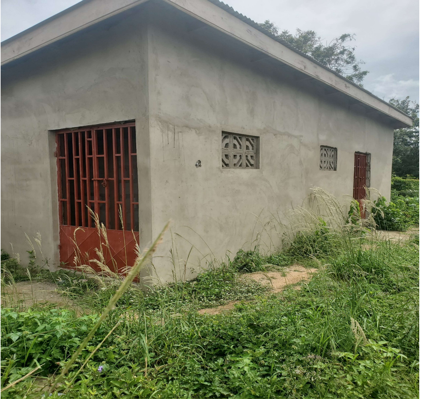
Figure 5: 1 No. 4-Seater WC & 2 No. Urinal at Elmina Junction Lorry Park
